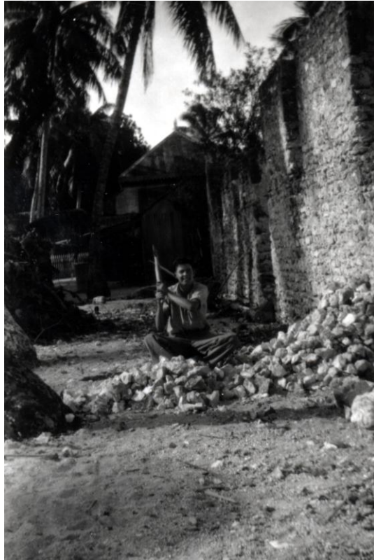
Elder Johnson breaking up coral rocks for the lime pit Jan 20 1936
