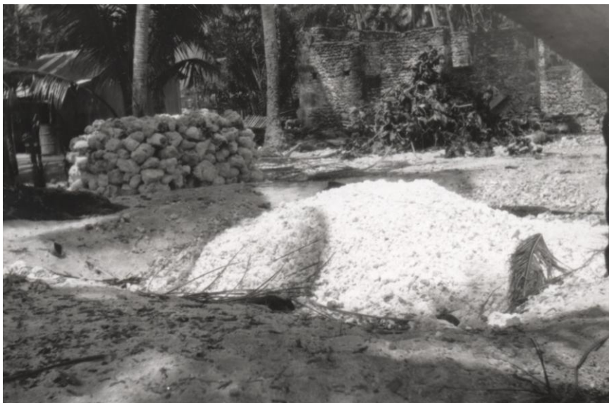
After five days of burning we have a good pile of lime for building the chapel. Sand is added to the lime to make a strong cement.
