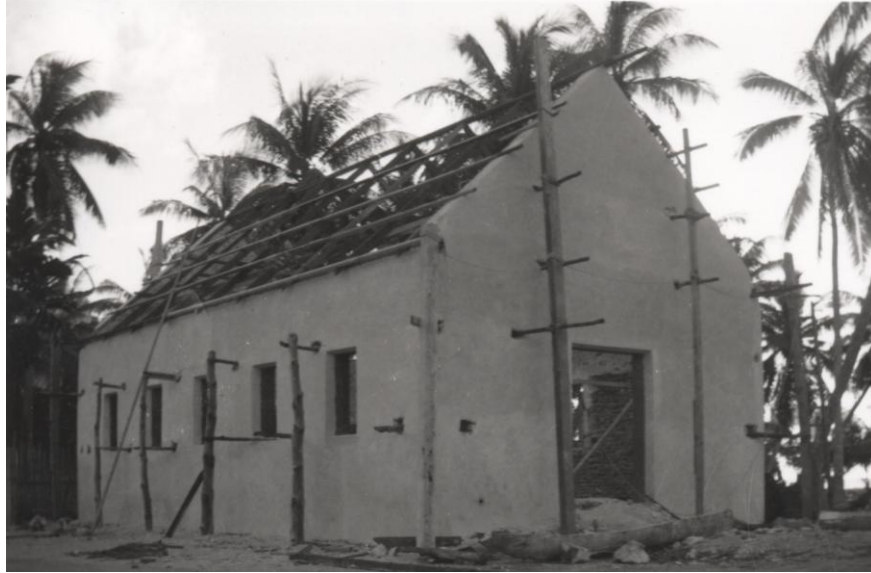
Putting the roof on. Elder Johnson had a miraculous experience of being saved from a fall from the roof.
