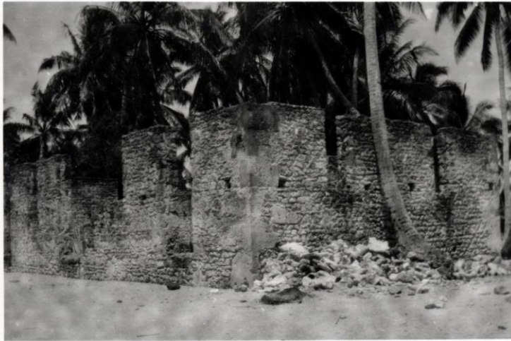
Picture of the old foundation before the renovation
