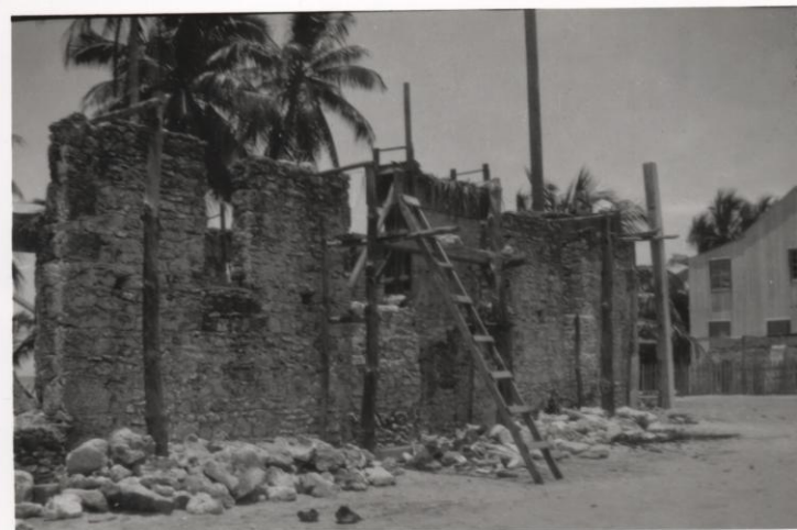
Getting the old foundation prepared for adding on to it
