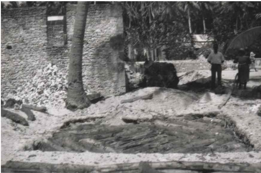
Laying the logs criss cross in the pit. It is built up about 3 feet above the ground and then the small rocks are put on top of the wood
