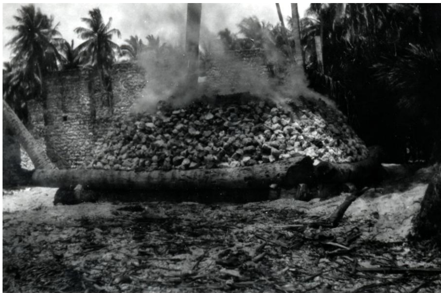
The lime pit has been lit and will burn for about five days.
