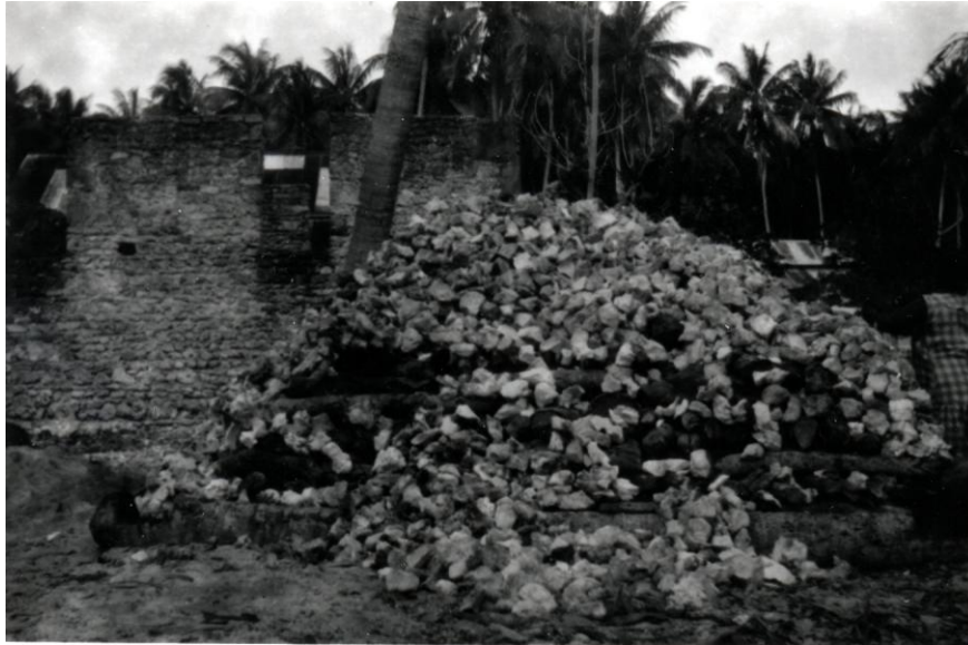
The lime pit with the lime rock being put on the logs to be burned. A whole is left in the middle of the rock and wood to pour kerosene into the bottom for lighting the wood.
